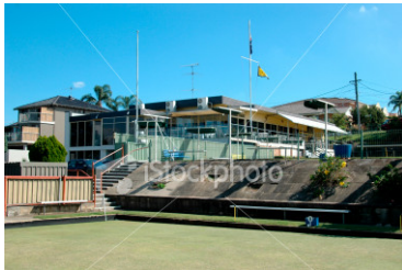
Sheltered Viewing Gallery Area
